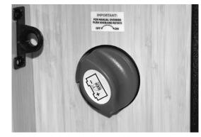
Push knob in before manually rotating it to the ON, OFF, or DISABLE function.
