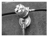
All models are equipped with a two-stage automatic change-over gas regulator that offers the convenience of automatic changeover from empty to full gas cylinders. Both tanks are connected to this regulator.
