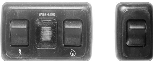
Two switch panels are located on the bathroom wall. The first switch panel, with a single switch, controls the lavatory lights. The second switch panel, with two switches and a red indicator, is for lighting the water heater.
