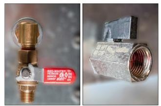
The fresh water line and tank drain valves are on the trailer's exterior for easier access. Between the tires, you will see a galvanized steel box a few inches lower than the trailer frame. The two brass valves are line drains. The stainless steel valve is for draining the fresh water tank.
