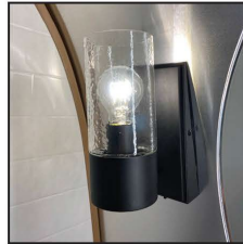
Bath Sconce Lighting: 513928 Custom developed to 12V for PB lavy MNF: Dave Carter Where: Mounted on aluminum, both sides of 20" round mirror in lavy
